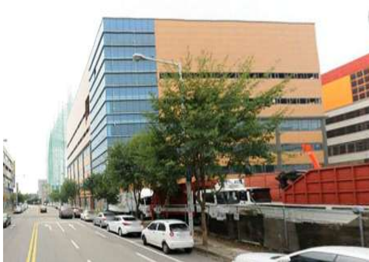
<Fig. 1> The abandoned building
